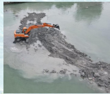
Work has started at English River project
