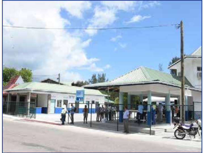
Cascade fisheries facilities. Photo Courtesy Seychelles Nation
