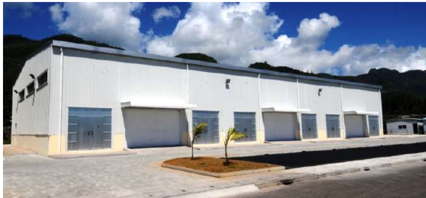
Figure 7.3 Providence fish processing factory
